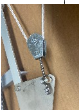
adjustment pulley for optimal window closing
