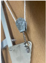
adjustment pulley for optimal window closing
