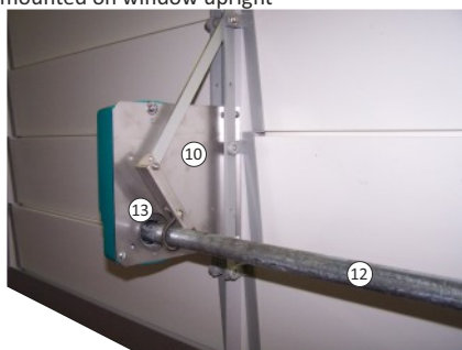
Detail of servomotor JOV.24V. mounted on window upright
